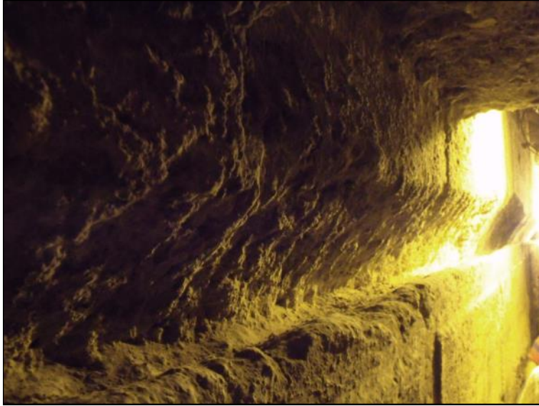
This channel was cut in the stone wall to serve as an aqueduct.
