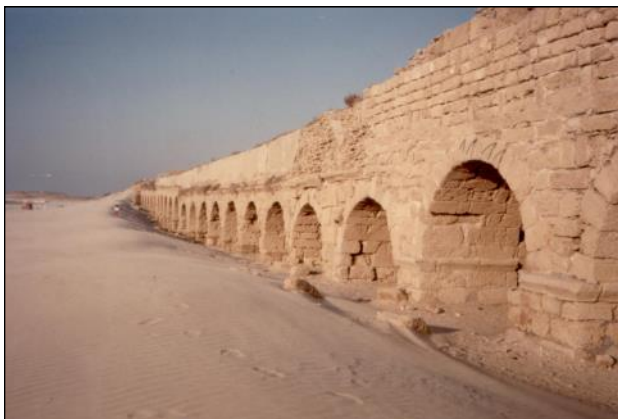
High Level Aqueduct Along the Coast
