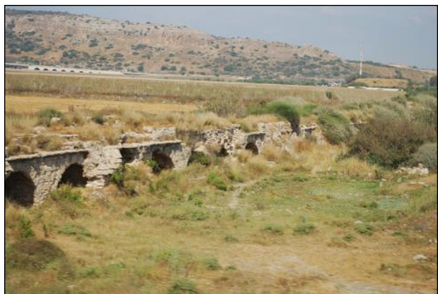
High Level Aqueduct from the East
