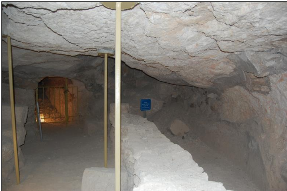
Tunnel and Water Inlet
