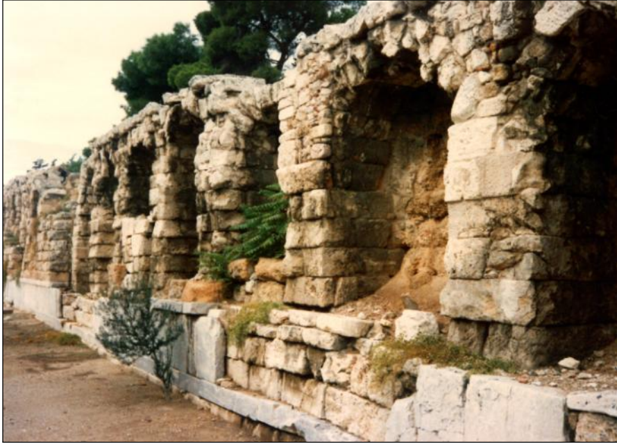
The Stoa of Eumenes was built at the southern base of the Acropolis in Athens. It was donated by Eumenes II, the king of Pergamum (197-159 B.C.).
