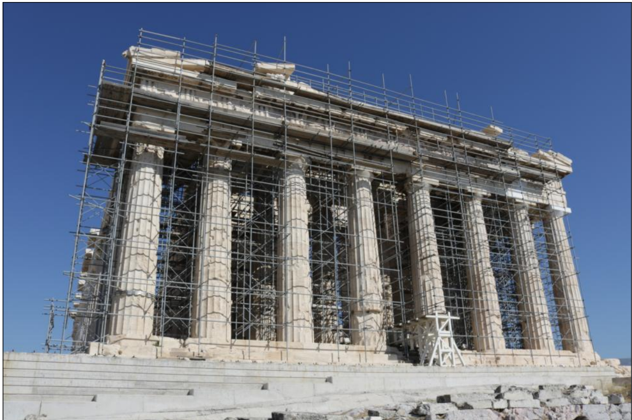
Restoration on the West Side of the Parthenon
