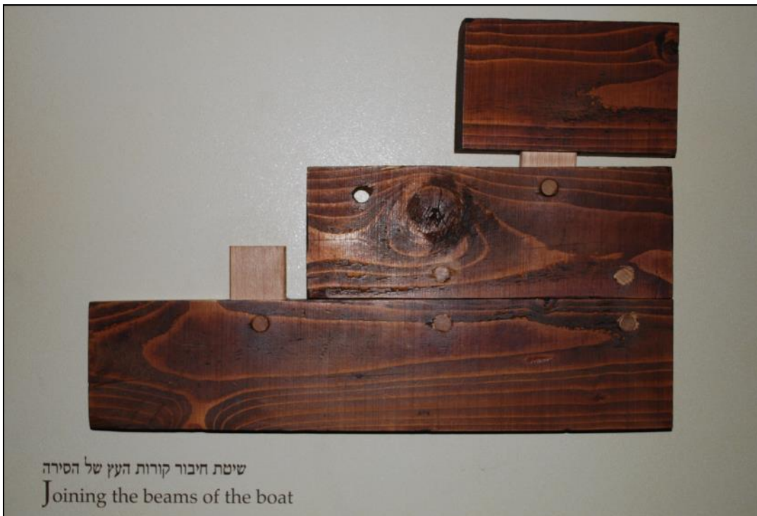
Mortise and Tenon Method Illustrated
